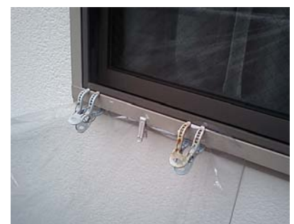
Clips attaching plastic sheet to a window frame
