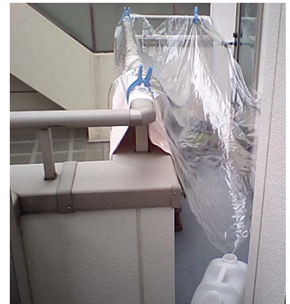
The installed system
